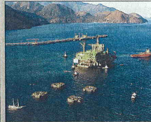
Step 4: Positioning the deck box above the submerged lower hull
