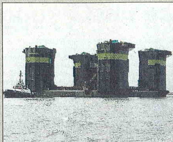
Step 1: Towing the lower hull in preparation for its mating with the P-52 rig deck
