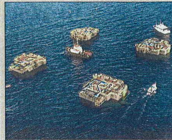
Step 2: Submerging the lower hull until only the upper ends of its four columns are above water
