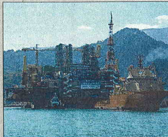
Step 3: Towing the P-52 deck box for mating with the submerged lower hull
