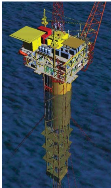
Figure 1. A truss spar has been a traditional deepwater option with heave plates to minimize platform heave at sea. (All graphics courtesy of FloaTEC LLC)
