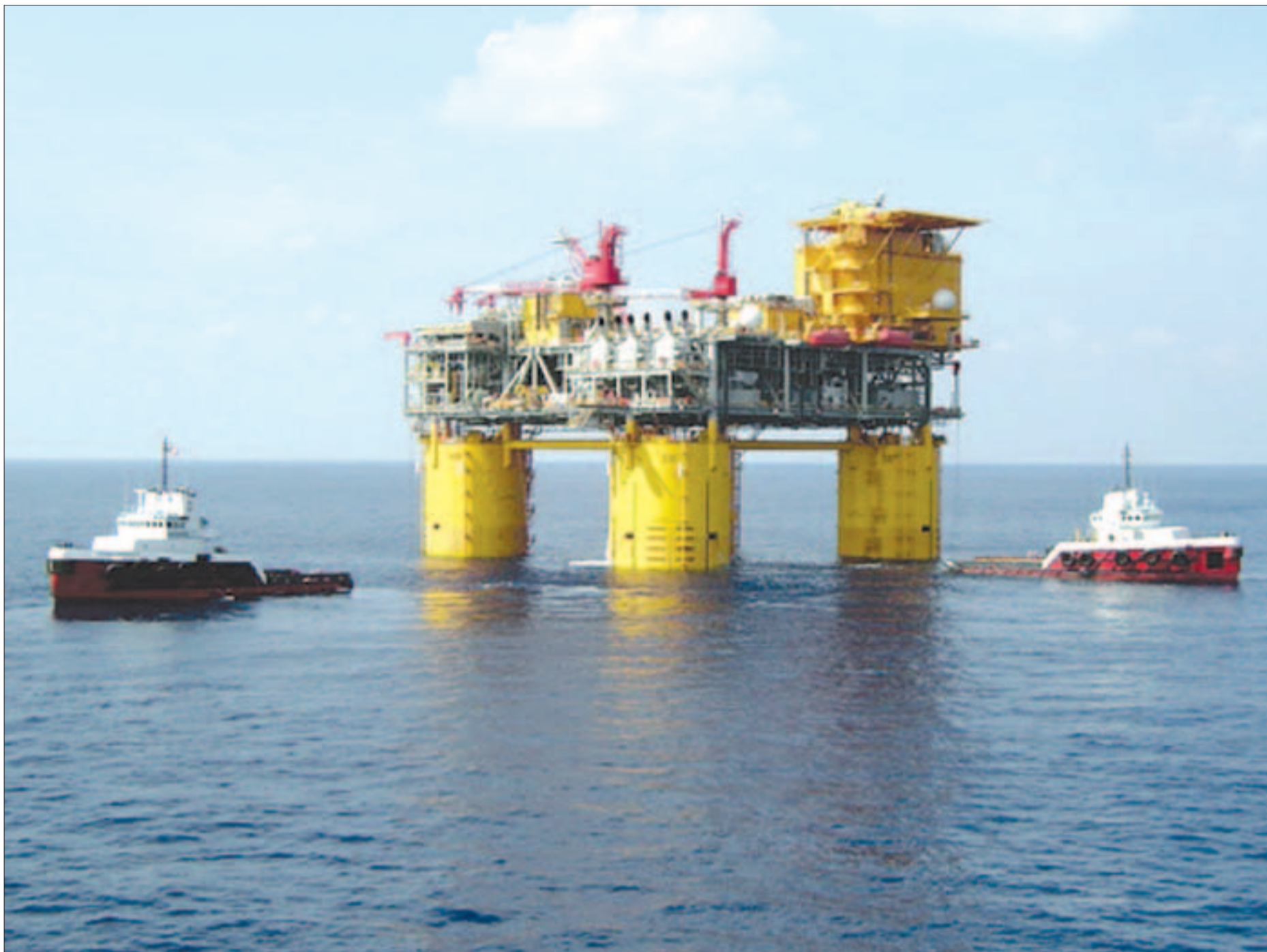
First run-out in Gulf: Conoco used the ETL design, then owned by ABB, for its Magnolia oil production platform (above) Photo: NOAA
